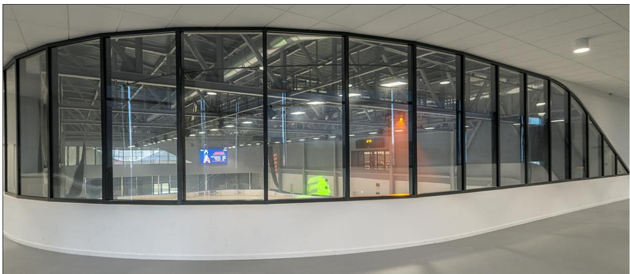
Working closely with the Pyroguard technical team, Pyroguard T-EI60 from the Pyroguard Protect range, was chosen for its ability to be custom manufactured to suit the individual project's needs. The Pyroguard toughened fire safety glass provides 60 minutes of protection against flames and smoke and enables the transmission of natural light, acoustic control and thermal and solar performance, while losing no aesthetic benefits and maintaining the highest standards of safety.
