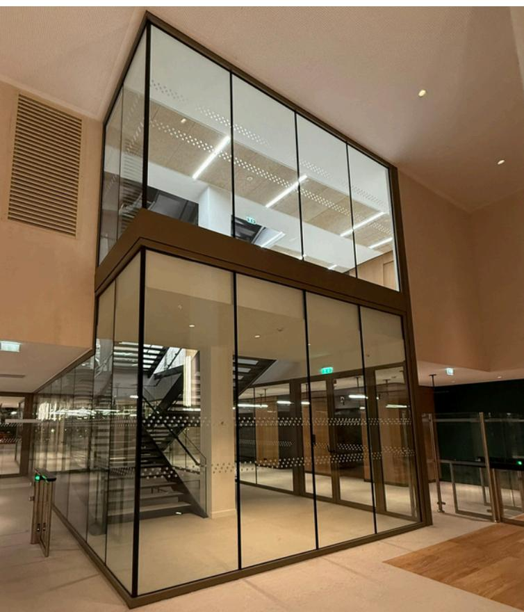
To support the architects' vision of light and openness, 650 m<sup>2</sup> of Pyroguard Protect EI60 fire-rated glass was installed internally to form elegant edge-to-edge partitions around the stairwells, atrium and meeting rooms to provide visual continuity while meeting vigorous fire safety standards.
