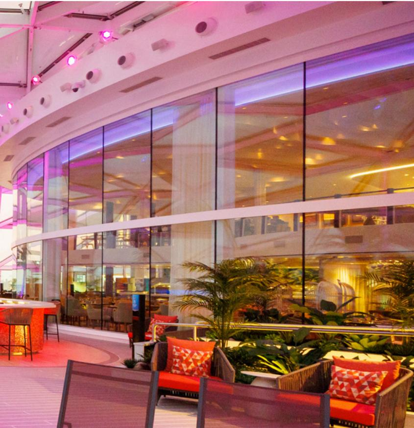
The system was tested to ensure that it met the required fire safety standards for the marine environment. The testing was carried out by the accredited test laboratory Efectis in France. To meet the A60 class requirement, the system must withstand flame for 60 minutes without catching fire on the unexposed side. The system successfully achieved an A60 class rating for straight walls and an A30 class rating for faceted walls.
