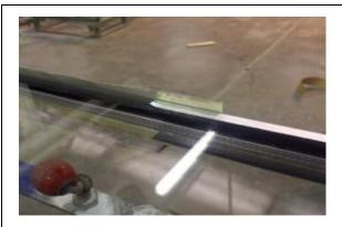
The ends of the PAL tape must overlap by a minimum of 40 mm on the upper third of the height of one of the side edges.
