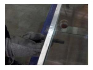
Flip the glass, taking care to respect manual handling rules. The PAL tape is then pressed onto the bottom face of the unit using the plastic smoothing tool.
