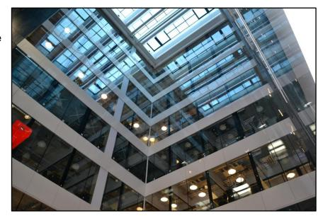
this aspect of the project in on time would be critical. As a result, Walls to Workstations (W2W) - who were tasked with removing and replacing the five-floor atrium – had just six weeks to see the project through to completion. Involving complete removal of the non-fire-rated glass and frame and installation of a new E30-rated system, W2W would rely on its delivery partners to bring the project in on time and to the highest standards of quality.
